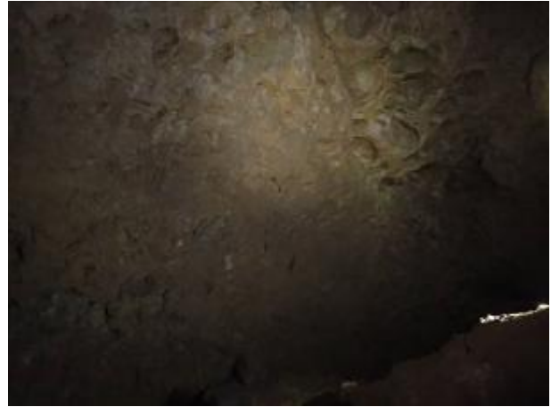
Phreatic evidence on the roof
