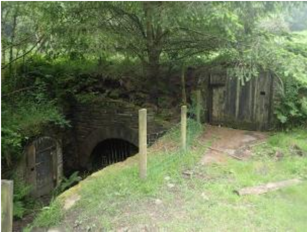
Morses Level. Cabin to left and compressor house to right
