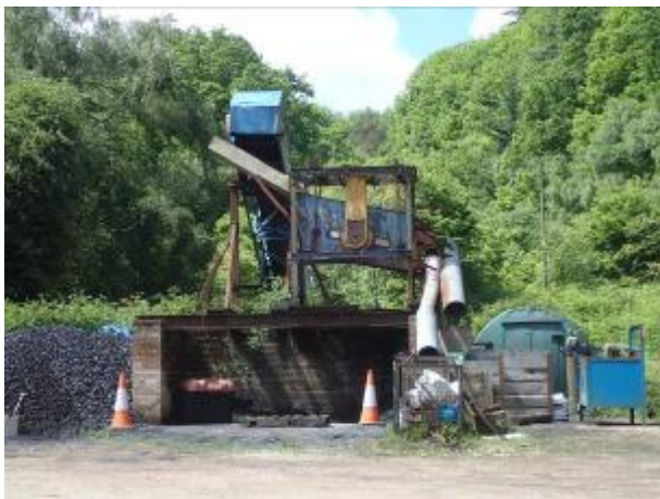
Hopewell coal processing plant
