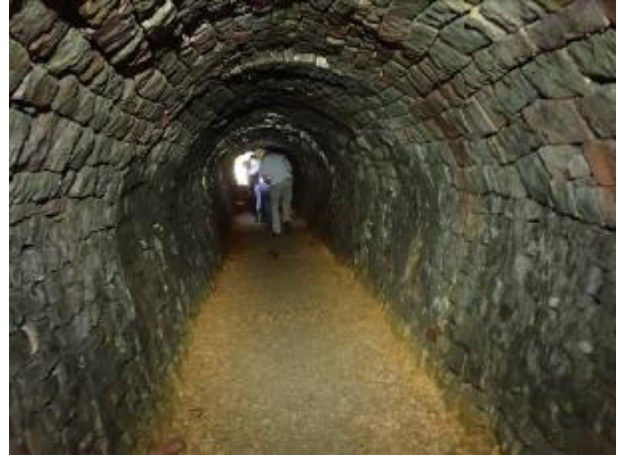
The last section of the adit
