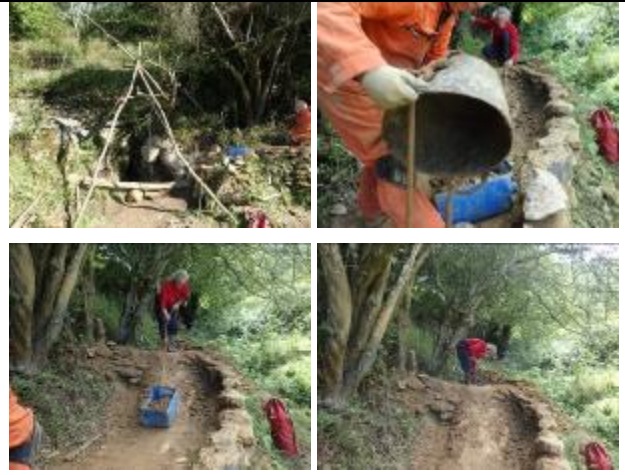
The digging system: (1) bucket raised, (2) bucket emptied, (3) spoil dragged away, (4) spoil dumped. Note the Egyptian-style ramp.
